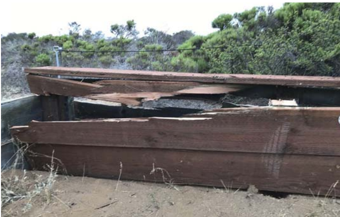
16th Street Parking area backstop, heavily damaged when a truck crashed into it. The damage was promptly repaired by County Park Rangers. Photo by Jay Waddell.
