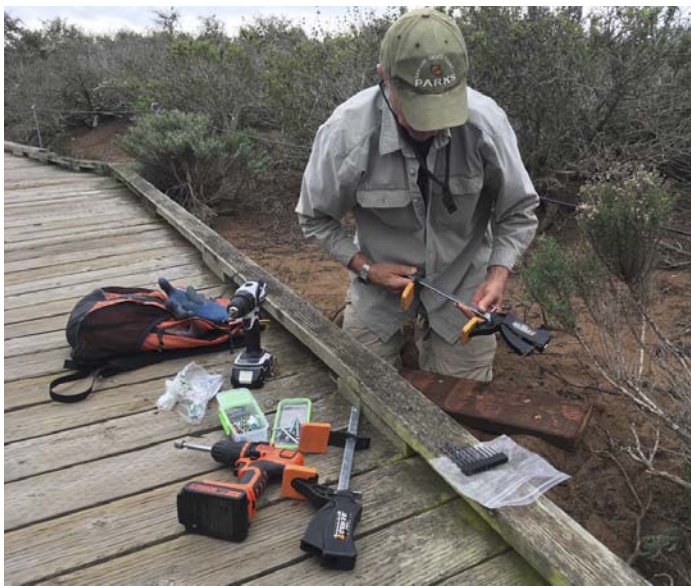
During the March SWAP work party, Rich Johnson replaced a broken boardwalk stringer. Photo by Prisila Johnson.
