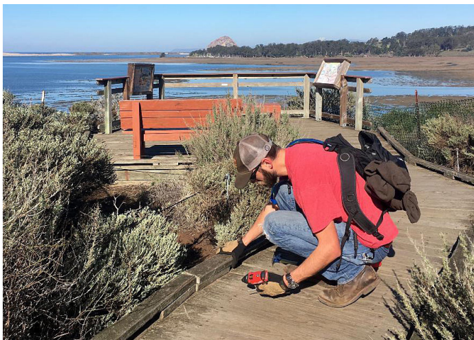
Weed Warrior Drew Bentz repaired a broken boardwalk toe rail during February's work party. Photo by Rich Johnson.
