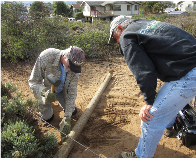
During the December 2nd work party, Dean Thompson (left) and Skip Rotstein moved a peeler log water bar on the 17th Street path to a place where it would be more effective. Photo by Yolanda Waddell.
