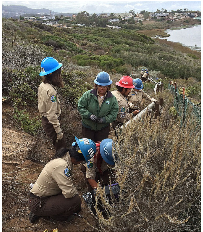
A deteriorating wood rail fence that was no longer needed was removed by CCC crewmembers as part of the Bush Lupine erosion control project. Photo by Skip Rotstein.
