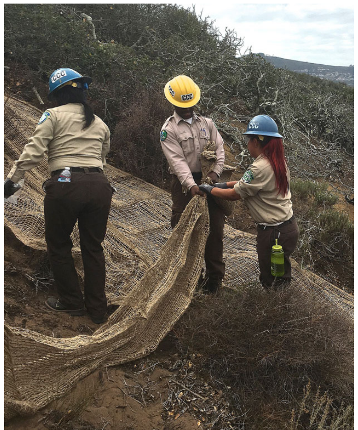
CCC crewmembers placed jute netting on a steep sandy hillside next to the Bush Lupine Point observation deck. Photo by Barrett Holland.
