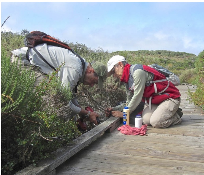
Weed Warriors Rich and Prisila Johnson fasten a section of boardwalk railing that has come loose. Photo by Yolanda Waddell.
