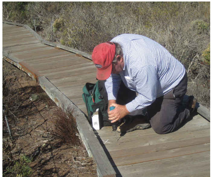
During the October work party Weed Warrior Jack Fanselow installs a stainless steel screw in a loose boardwalk board.
