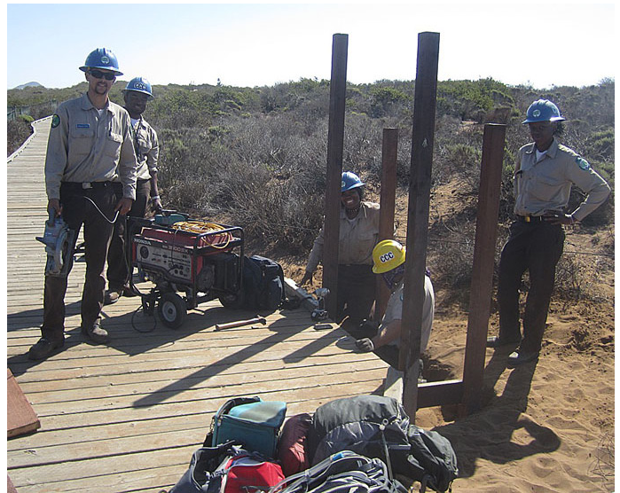
A CCC crew has removed the old steps, dug deep holes to install rail supports, and is preparing to build a new step next to the boardwalk at the 13th Street trail.
