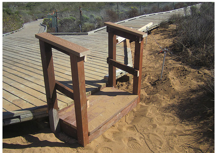
The finished step with plastic “wood” rails at 13th Street. Additional steps and rails were built at 14th, 15th and 17th Streets.
