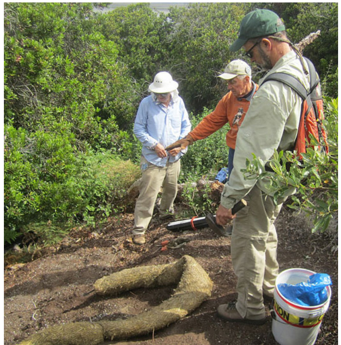
Ron Rasmussen (center) discusses with Dave Bowlus (left) and Rich Johnson (right) the procedure for installing straw wattles on a disturbed slope in the Elfin Forest.
