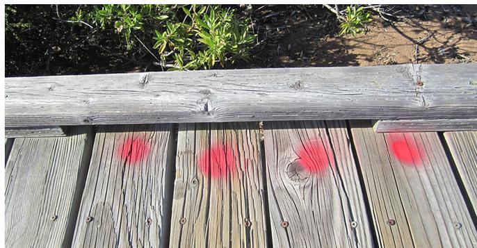
*Those four circles on boardwalk boards are just four of over 1,000 circles that Ron Rasmussen painted to mark boards that need to be replaced. Photo by Yolanda Waddell.*
