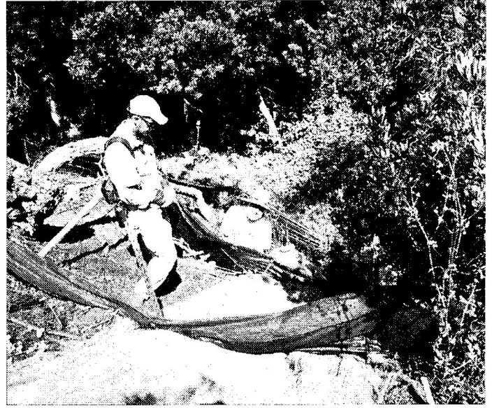
Rich Johnson, Pete Sarafian and Prisila Johnson (not shown), did some repair to silt fencing, including installing coconut fiber matting, during the July 4th work party. Photo by Yolanda Waddell.
