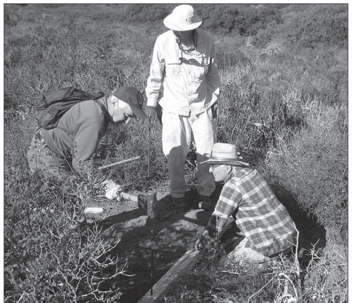
Ron Rasmussen, Conservation Chair Pete Sarafian, and Dave Bowlus install an erosion control board across a trail in the Elfin Forest.
