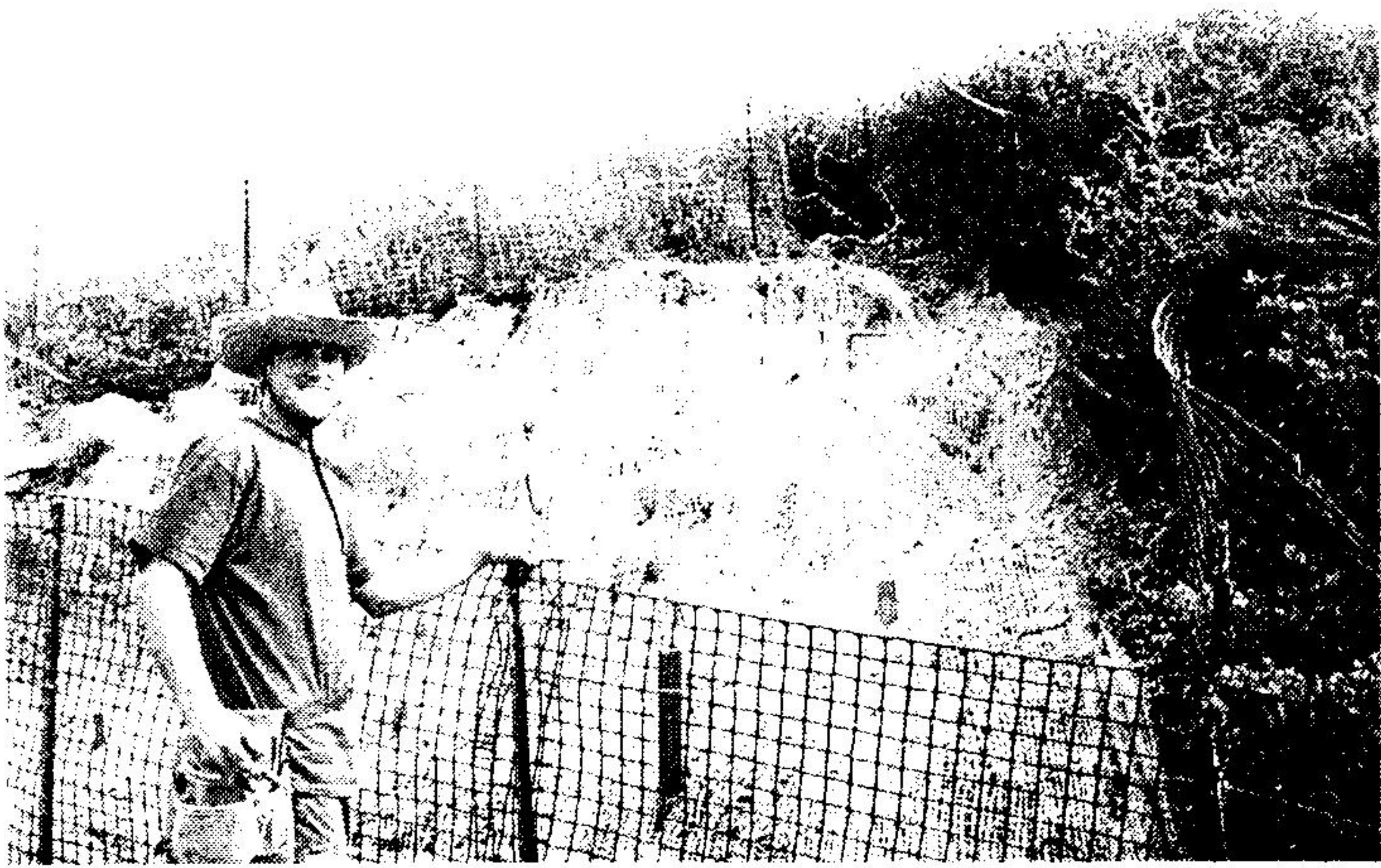
Josh Carmichael puts the finishing touches on his "jute taco," which will control erosion on the slope above Bush Lupine Point. Photo by Yolanda Waddell.
