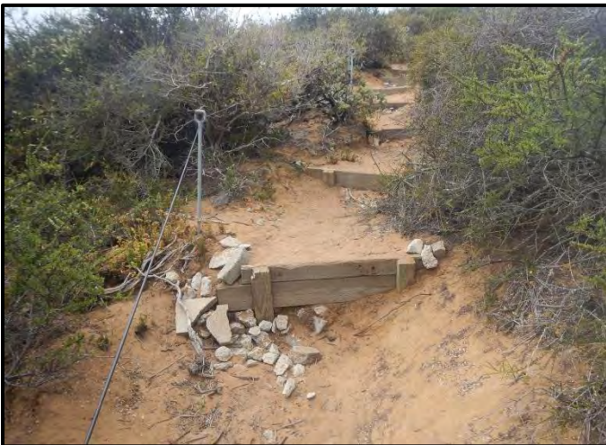
Photo 35. Grade control structures and concrete chunks on steep slope south of the Klopfer Grove (07-13-18).
