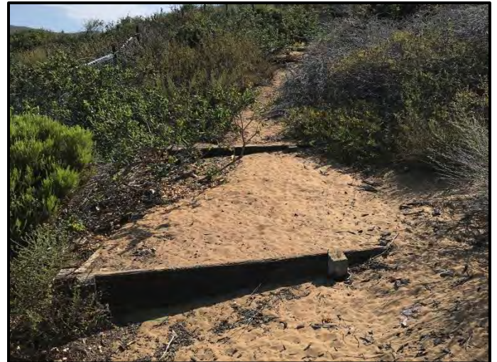
Photo 34. Wooden grade control structures employed on sand trails; Orchid Trail shown here (07-13-18).
