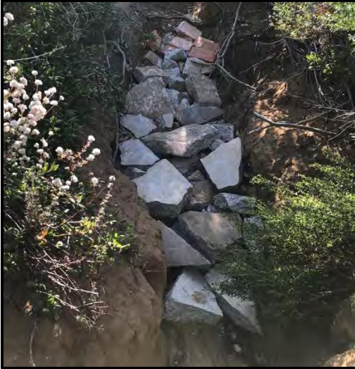
Photo 37. Deeply incised gully lined with large concrete chunks, west of 11 th Street trailhead (07-19-18).
