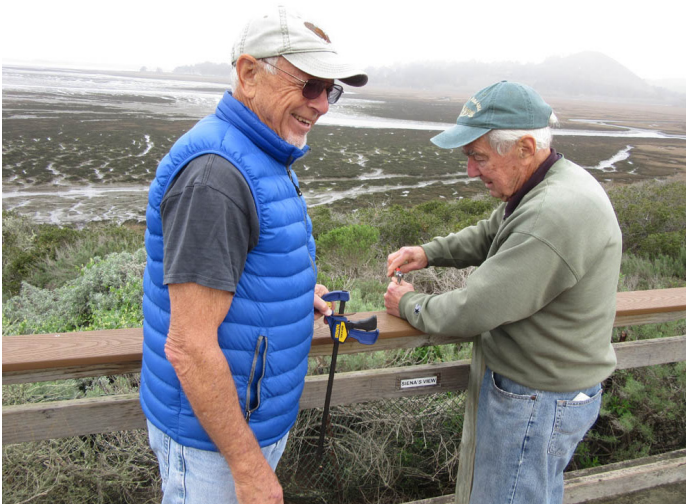
In February, Conservation Chair Skip Rotstein joined Ron Rasmussen in replacing a badly vandalized rail at Sienna’s View overlook. Photo by Yolanda Waddell.
