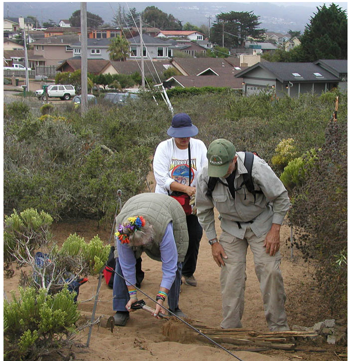
Replacing a decayed water bar on the 12th Street Trail during the September work party were (L-R) Lannie Erickson, Annette Kennedy and Rich Johnson.
