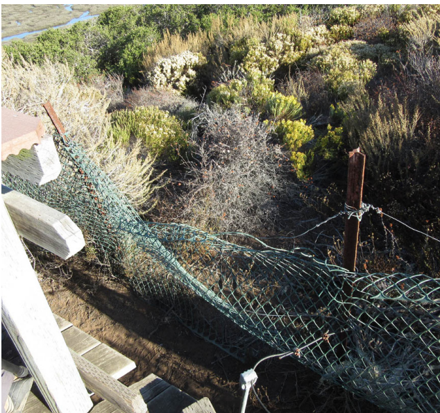
Someone objected to the presence of a fence at Siena’s View overlook and climbed over it, requiring it to be repaired. An “Elfin Forest Watcher” reported this to SWAP. Photo by Yolanda Waddell.
