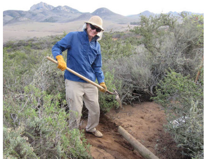
In preparation for El Niño, Dave Bowlus moves sand on a trail so that rainwater will flow away from the trail and onto land covered by vegetation. Photo by Yolanda Waddell.
