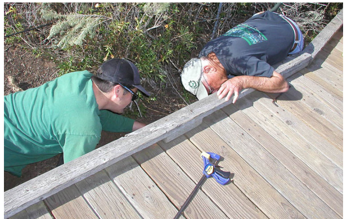
As the boardwalk ages, more things break. Working in April to replace a broken stringer, a board that holds up the boardwalk, were Barrett Holland (left) and Conservation Chair Skip Rotstein.
