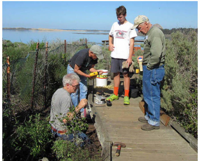
In March, some skilled carpentry was done to replace a broken boardwalk stringer by (L-R) Craig Johnsen, Skip Rotstein, Matt Ellingen and Ron Rasmussen.
