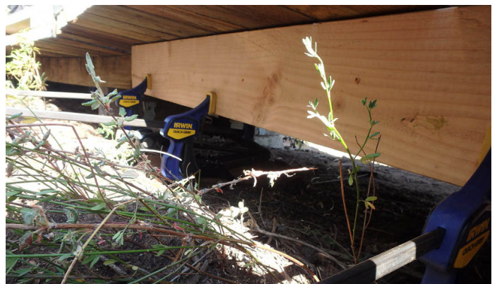
Shown is a replacement stringer board with clamps to hold it while glue dries. The boards are both nailed and glued to keep them firmly in place. Photo by Barrett Holland.
