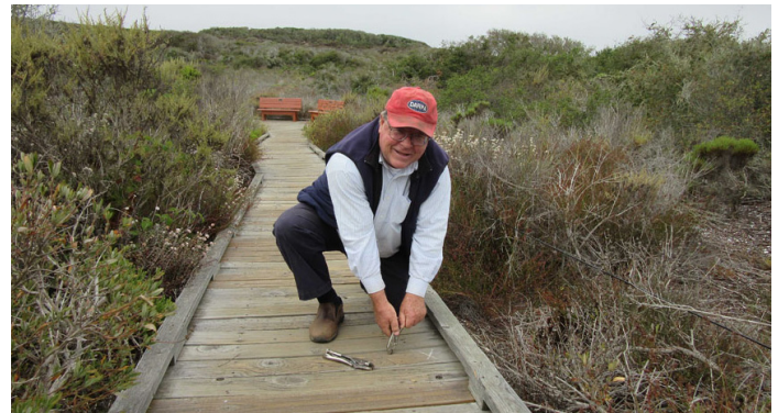
Weed Warrior Jack Fanselow spent the August work day doing boardwalk repair. His task was to remove old rusted screws from boards that had “popped up,” and replace them with stainless steel screws. Photo by Yolanda Waddell.
