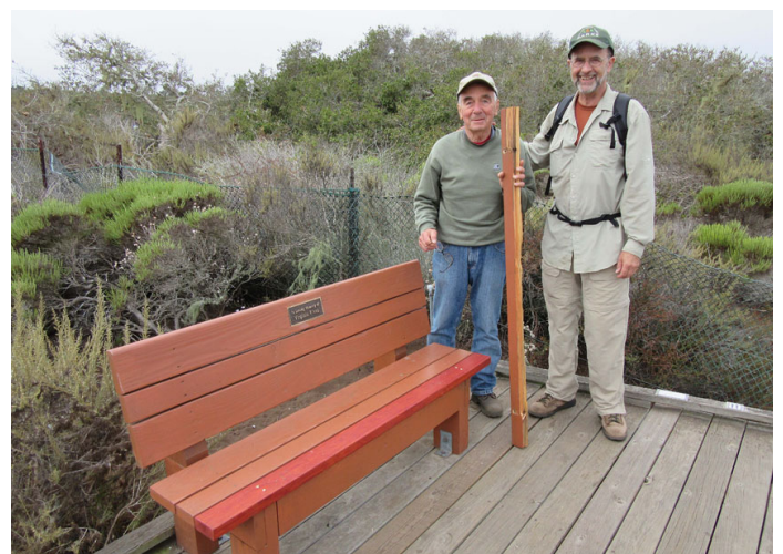
During the August work party Ron Rasmussen and Rich Johnson replace a mangled bench board (held by Ron) with a new one. The color doesn't quite match, but the bench is now comfortable.
